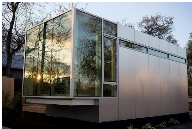
Picture 4. Modular house in high-tech style
